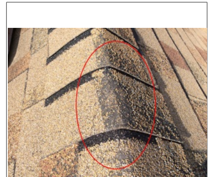
Photo of ridge cap showing significant loss of granules.
