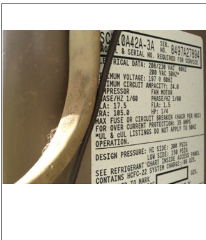
Improper wiring. Green wire is ground from satellite dish.
