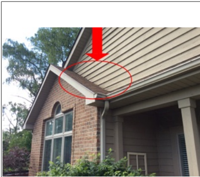
Wood siding showing deterioration.
