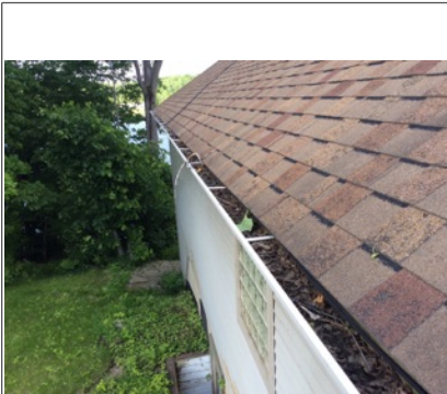
Photo showing debris in gutter. Recommend cleaning.
