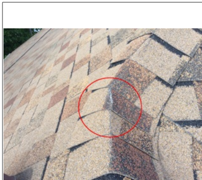
Ridge cap showing missing granules and cracking.
