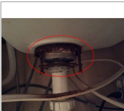
Photo showing corrosion of drain below sink.
